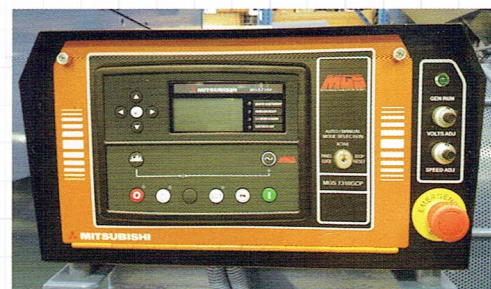
Alarms are indicated by an LCD and LED illumination.
